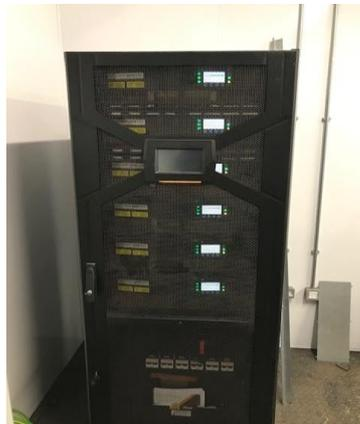
The PowerWAVE 9250DPA is a true modular uninterruptible power supply, scalable from 50kW up to 1.5MW, for power applications in critical, high density computing environments, such as pharmaceutical facilities.
